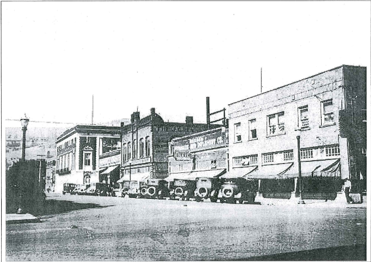
Depot Street, c. 1927, looking southwest from Adams Avenue. Observe the original lampposts and awnings. Contrast the changes in the building facades to the existing storefronts.
