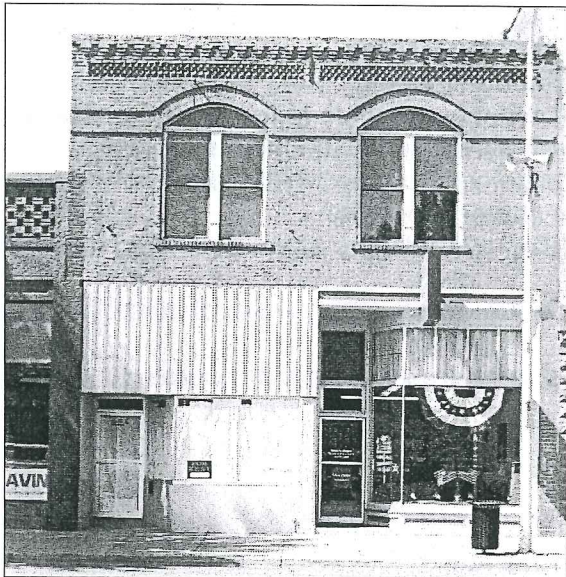
This building exhibits an original storefront on right with alterations occurring at the left.
