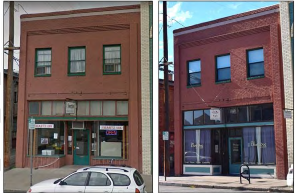
212 Fir Street is a good example of a rehabilitated storefront. Note the new pannelized bulkhead beneath the storefront windows. (Source for image on left:
