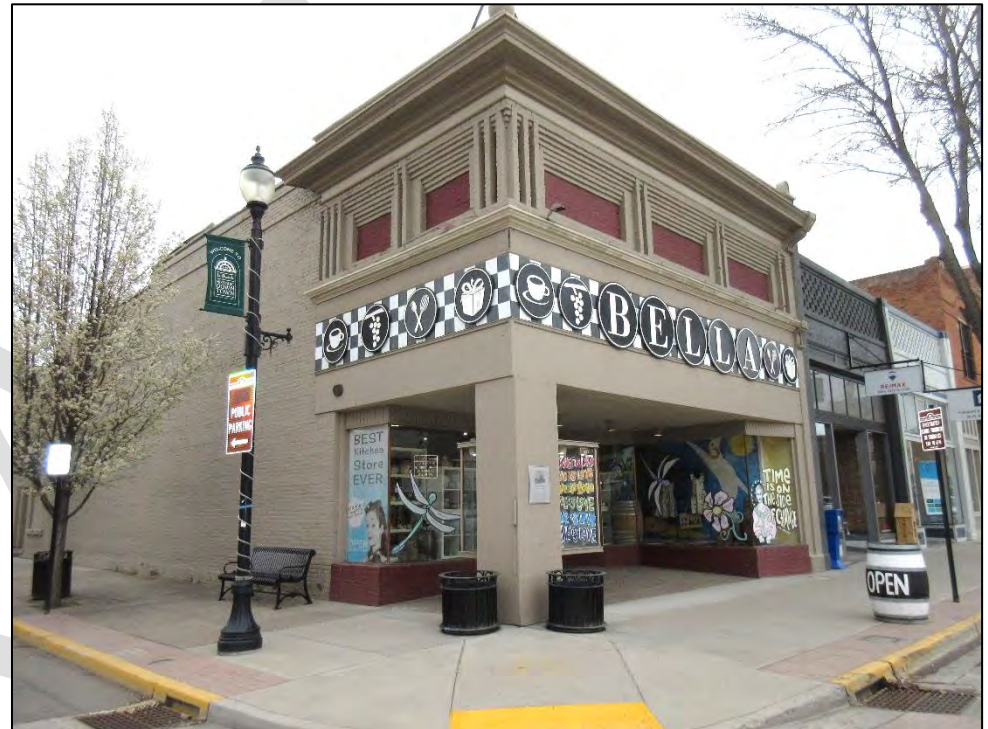
A way to retain the historic column and bay structure and introduce a modern storefront with ADA ramp. Everyone uses the same sloped entry.
