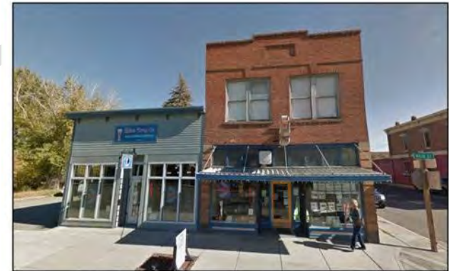
Example of a modern addition made to look like a separate building that fits in with surrounding historic buildings. Wright's Drug Store Building (105 N Main Street, Union, Oregon) (Source: Google Streetview 2012 and 2018)
