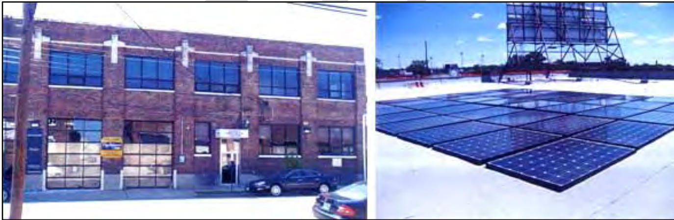
Using flat or low-slope solar panels is a simple way to limit visibility. (Sources: National Park Service: https://www.nps.gov/tps/sustainability/new-technology/solar-on-historic.htm )
