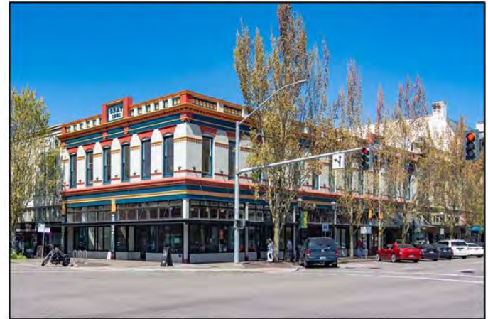
Gray Building (105-135 Liberty Street NE, Salem, OR) Rehabilitation of historic awning configuration from circa 1912. (Source: Willamette Heritage Center, Google Streetview 2012, City of Salem)
