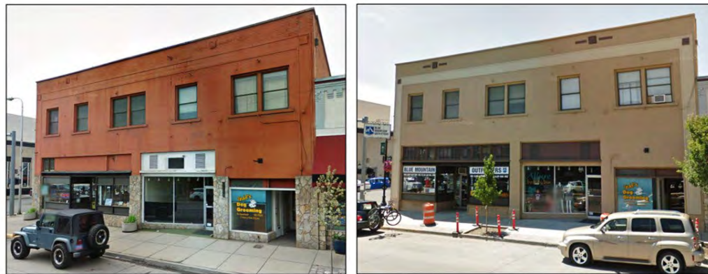
Ralston Block (1124 Adams Avenue) Note the removal of the added “fieldstone” facing and restoration of the historic painted brick wall finish. (Source: Google Street View 2012 and 2015)
