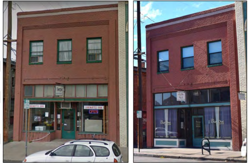
212 Fir Street is a good example of a rehabilitated storefront. Note the new paneled bulkhead beneath the storefront windows. (Source for image on left.)
