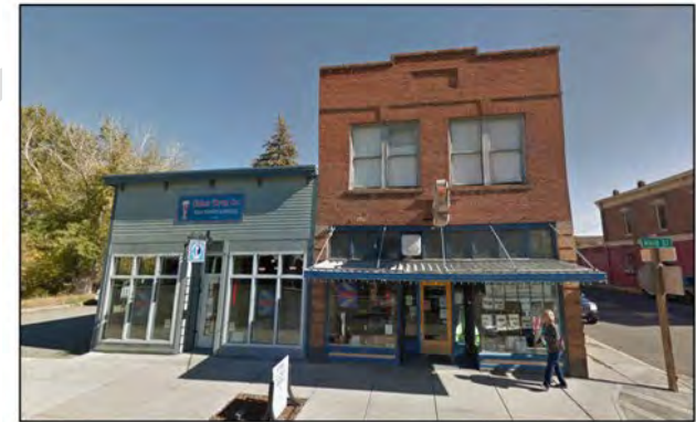
Example of a modern addition made to look like a separate building that fits in with surrounding historic buildings. Wright's Drug Store Building (105 N Main Street, Union, Oregon) (Source: Google Streetview 2012 and 2018)
