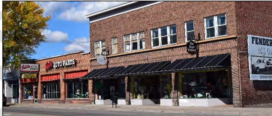
A variety of sign types are visible in this image, including blade signs, mounted wall signs, and internally illuminated letter signs. All are placed for pedestrian use and are no larger than historic building features at the ground level.
