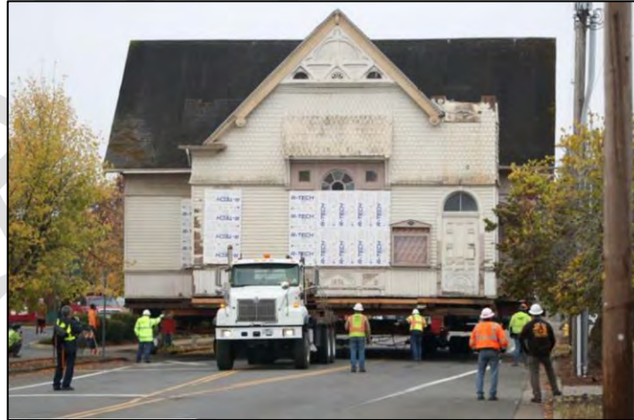
The historic Cumberland Church in Albany, Oregon, en route to its new location. The steeple was temporarily removed to facilitate the move. (Source: Corvallis Gazette-Times photo, October 2021)
