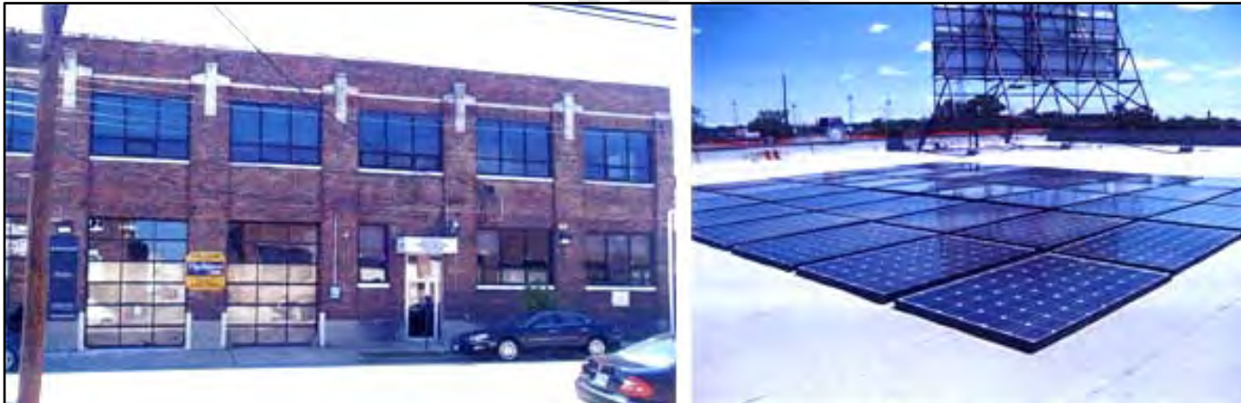
Using flat or low-slope solar panels is a simple way to limit visibility. (Sources: National Park Service: https://www.nps.gov/tps/sustainability/new-technology/solar-on-historic.htm )
