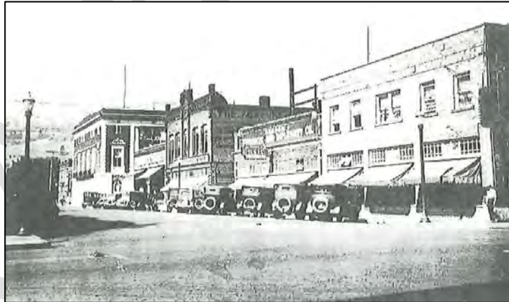
Depot Street, c. 1927, looking southwest from Adams Avenue.
