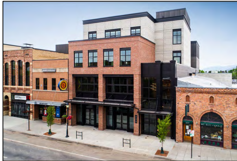
This infill development (2020) in Bozeman, MT created different volumes to break up the mass of new construction relative to the existing older buildings. The new building repairs and fills the gap in the streetwall. (Source: https://www.loopnet.com/Listin )
