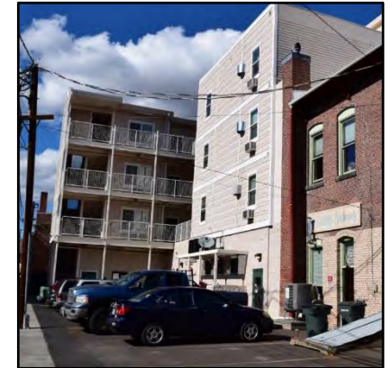
Example of materials that are allowable in the alley but would be unacceptable on the primary
