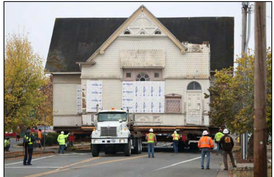
The historic Cumberland Church in Albany, Oregon, en route to its new location. The steeple was temporarily removed to facilitate the move. (Source: Corvallis Gazette-Times photo, October 2021)
