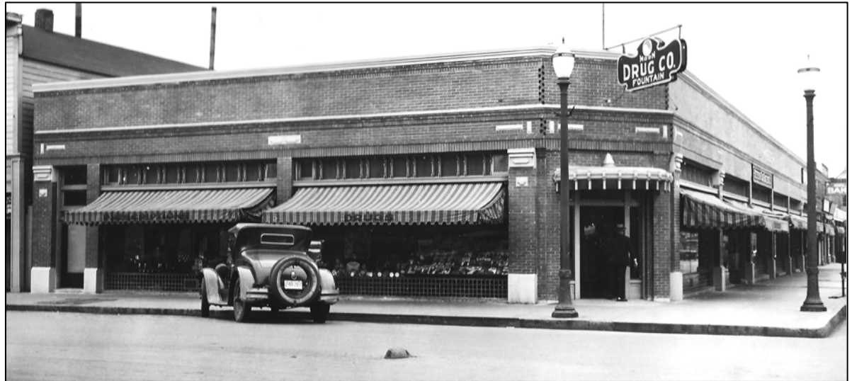
This circa 1930s image shows an ornamental canopy at the corner entry of the store, still present on the building. (Source: City of La Grande Archives)
