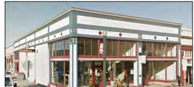
The Allen Building at 1004-1008 Commercial Street in Astoria, OR installed a historic inspired storefront. (Source: Circa 1920s Newspaper, 1989 Oregon SHPO Inventory Form, 2018 Google Streetview)
