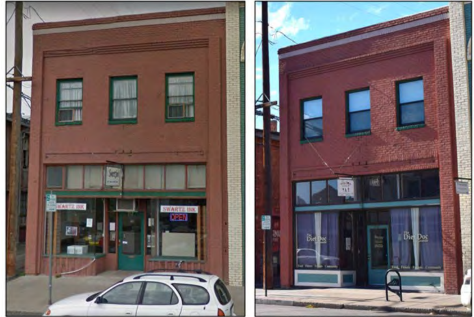
212 Fir Street is a good example of a rehabilitated storefront. Note the new panelized bulkhead beneath the storefront windows. (Source for image on left: Google Street View 2012)
