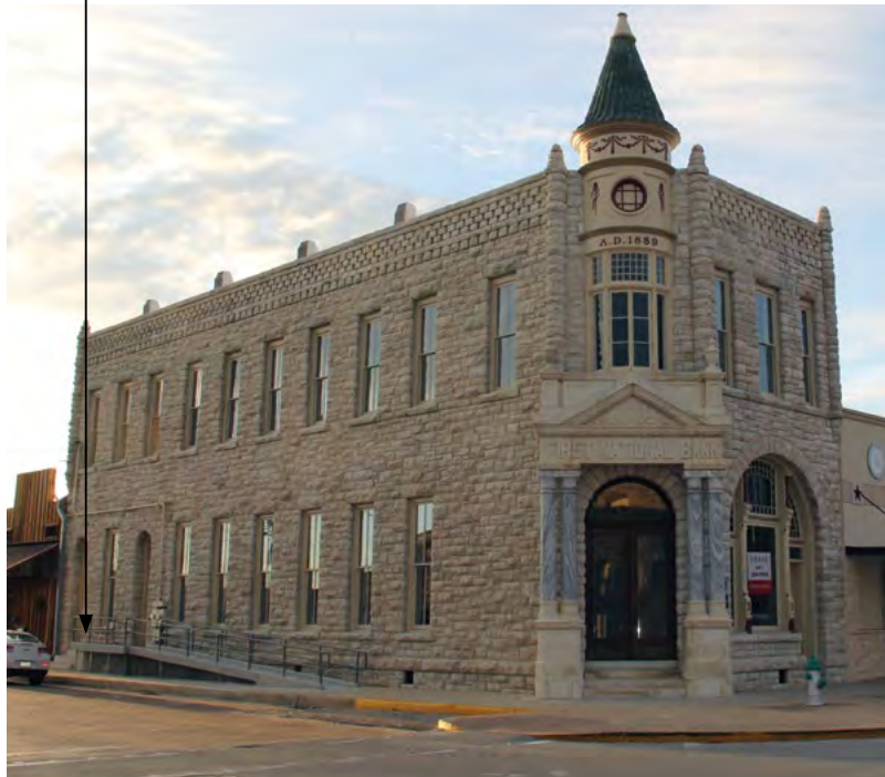
[53] This entrance ramp (right) is compatible with the historic character of this commercial building.
