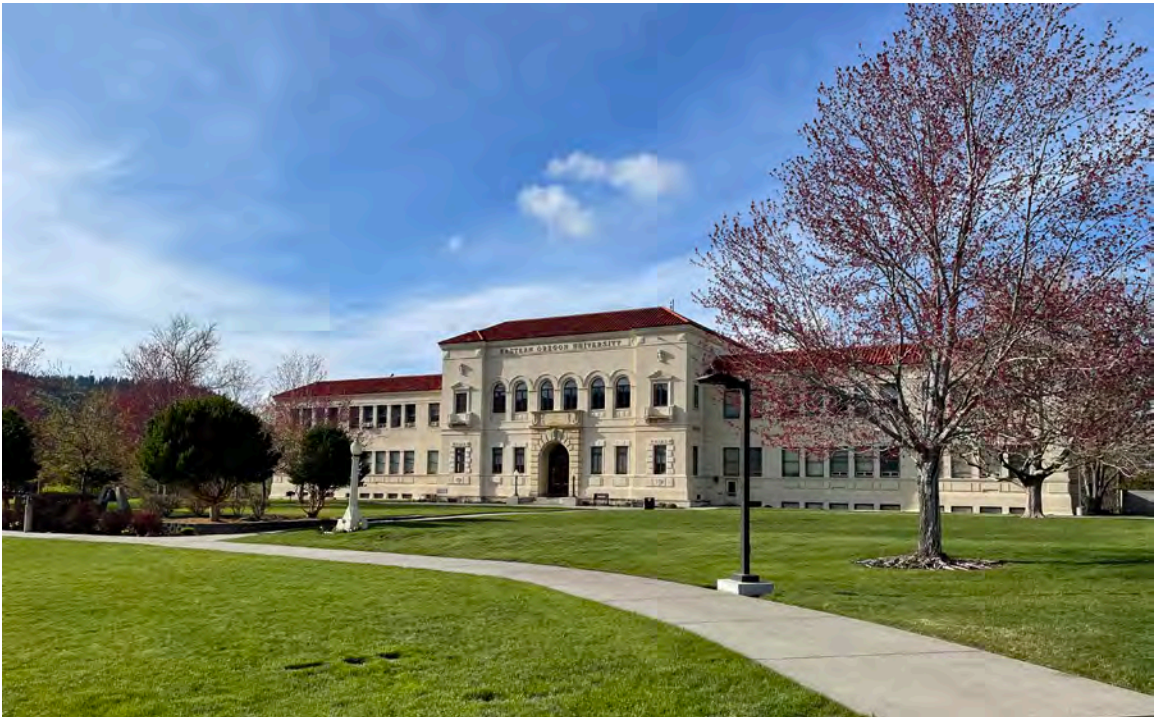
1. Inlow Hall south elevation, facing north. 04/12/2022.
