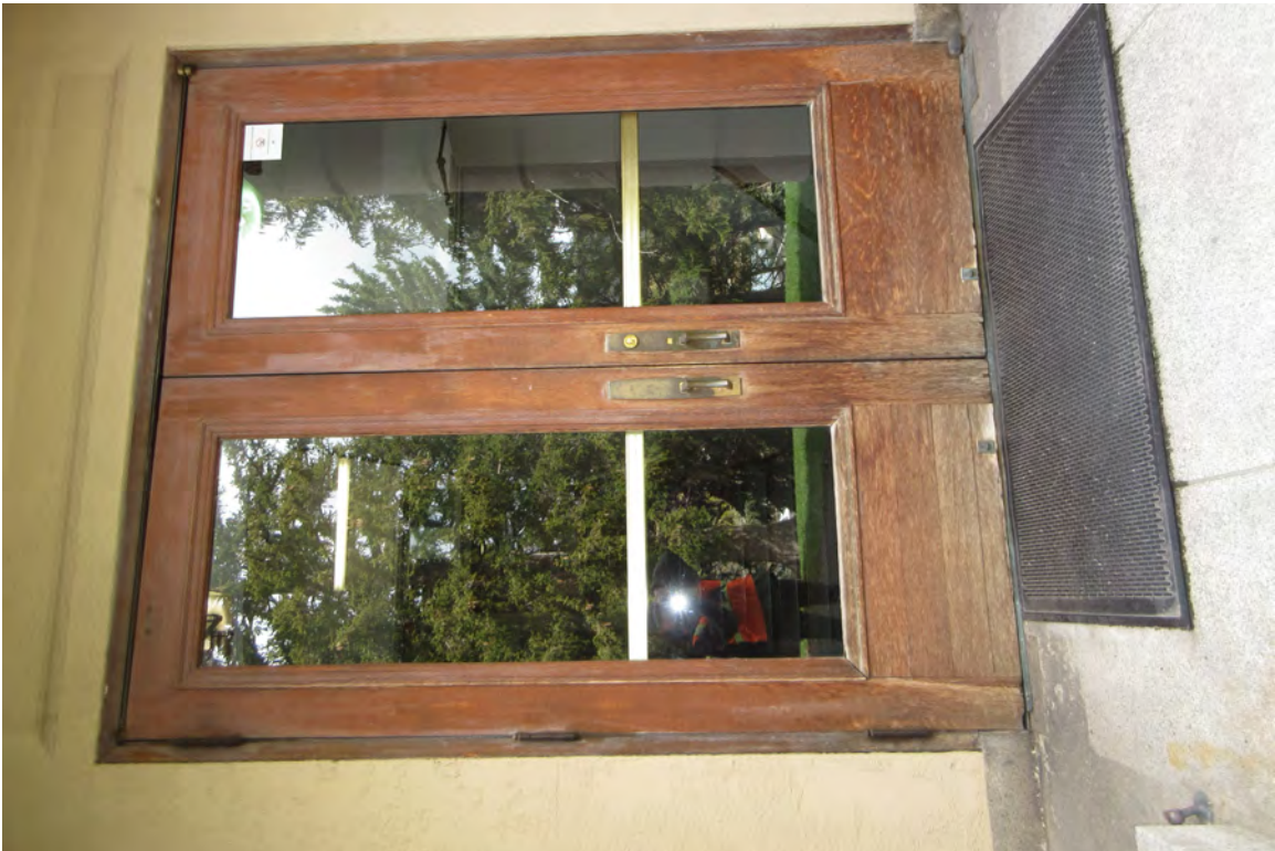
6. Example of primary entrance doors that will be refinished. 04/19/2022.
