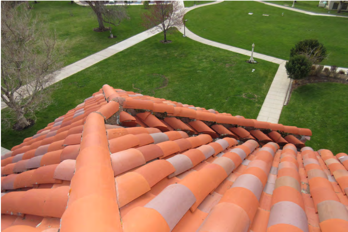
11. Example of terracotta roofing tile on southeastern corner of central pavilion roof, facing southeast. 04/19/2022.
