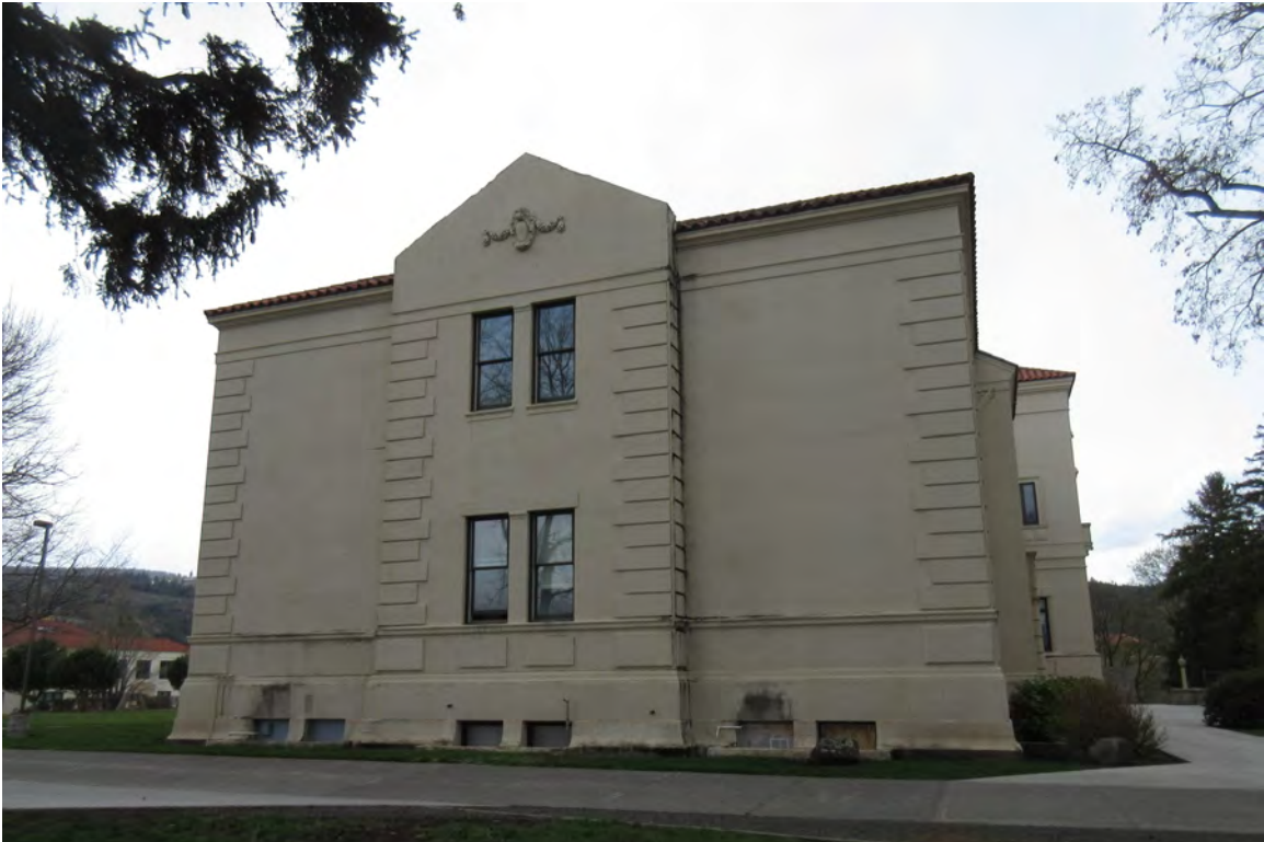
3. West elevation, facing east. 04/19/2022.
