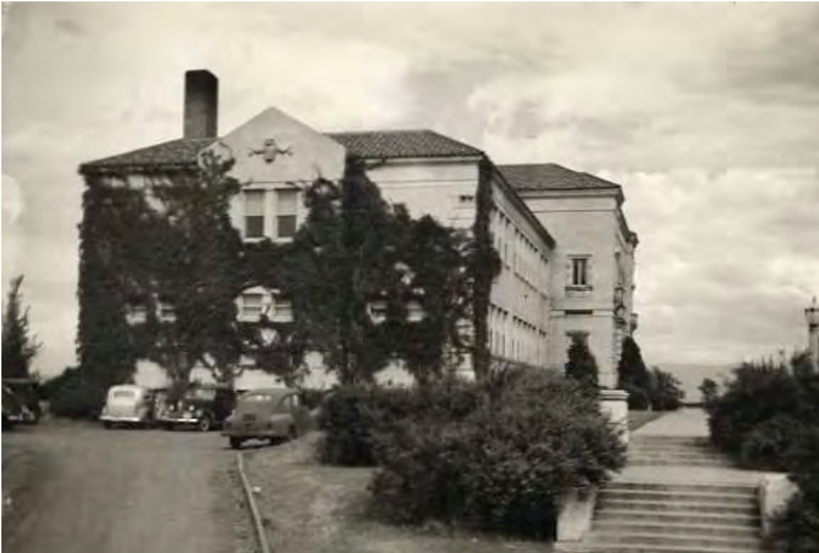
5. Inlow Hall, 1943. Southwest corner, facing northeast. Courtesy of Eastern Oregon University Digital Archives.
