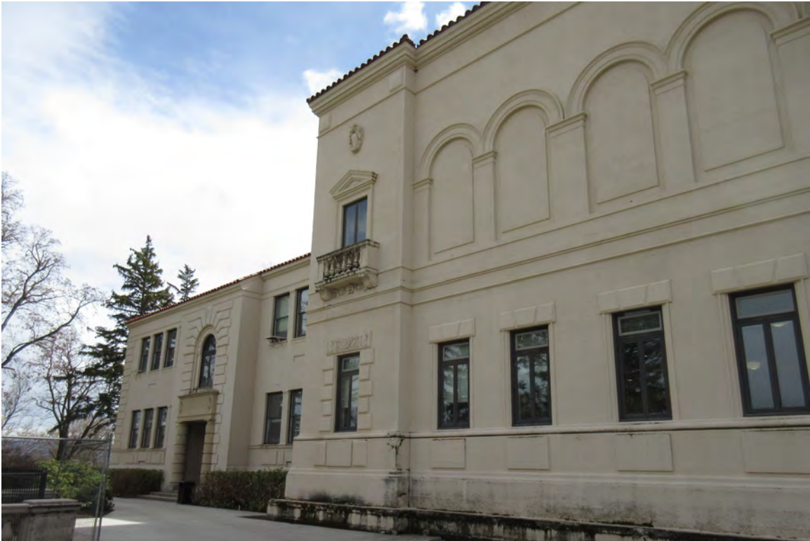
5. Western half of north elevation, facing southwest. 04/19/2022.
