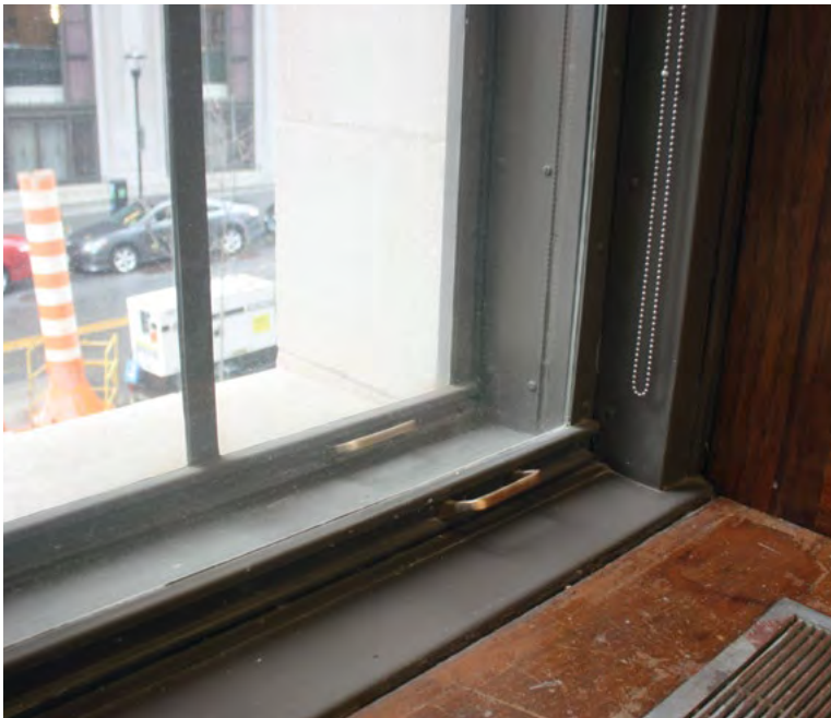
[18] The historic metal storm windows in this 1920s office building were retained and repaired during the rehabilitation project.
