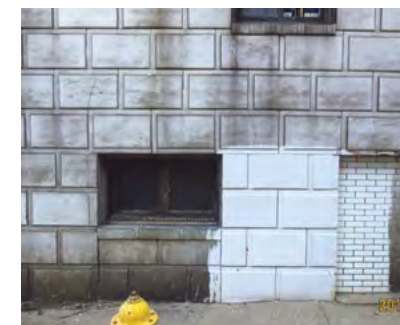
[1] A test patch should always be done before using a chemical cleaner to ensure that it will not damage historic masonry, as in this instance, terra cotta.
