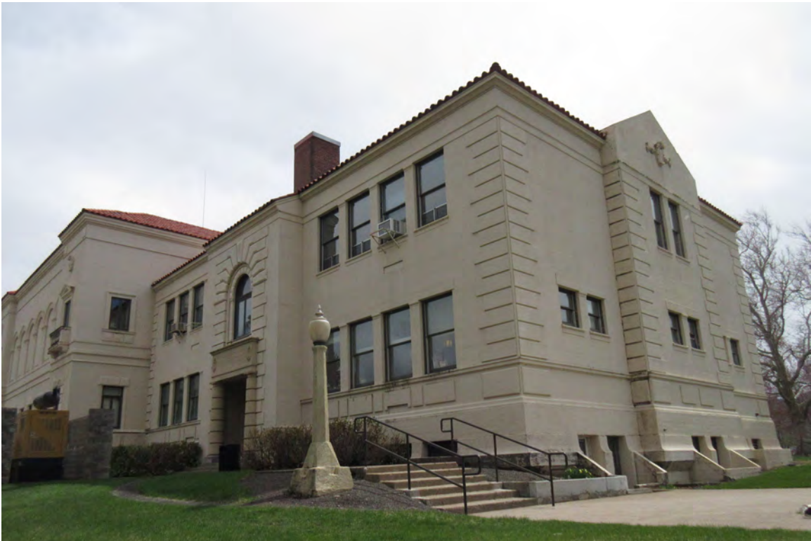
4. Northeast corner, facing southwest. 04/19/2022.
