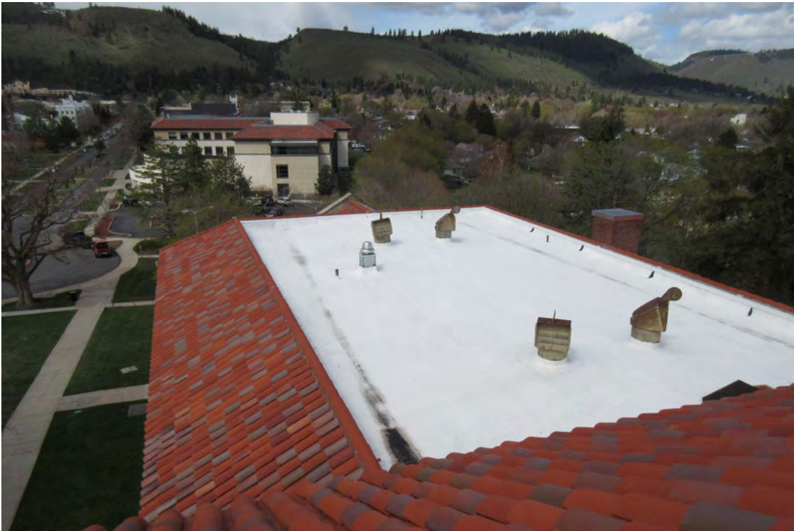
10. Inlow Hall's west wing roof. Terracotta tile and composite roof both to be replaced in kind. 04/19/2022..
