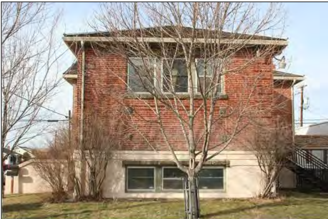
Photo 8 of 14: South façade, looking north.
