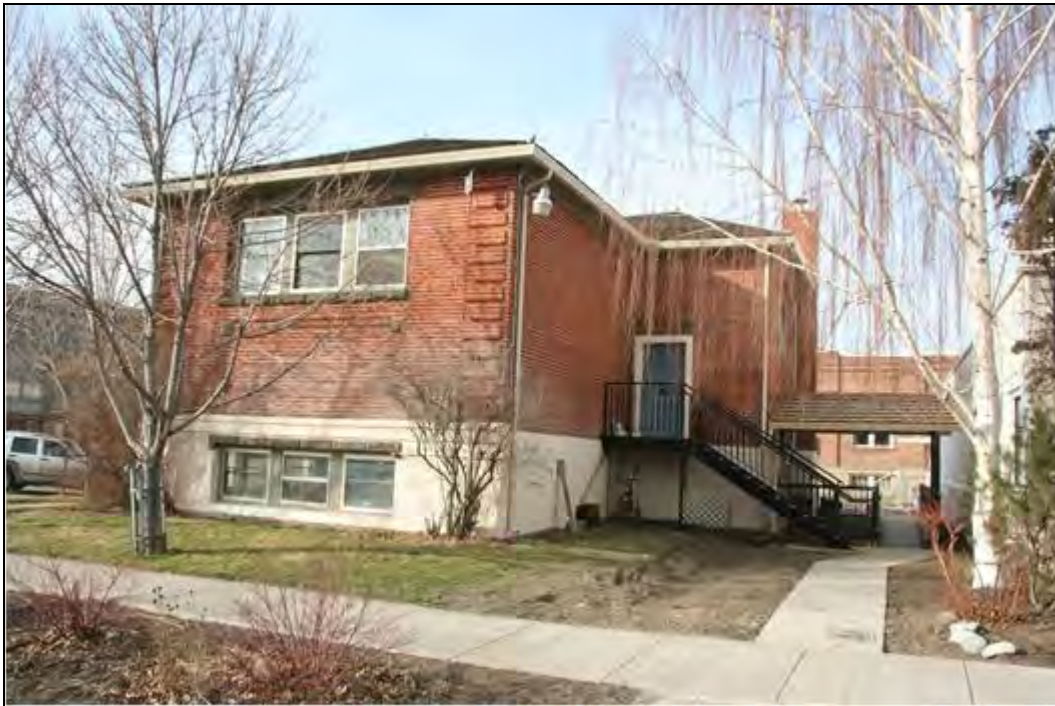
Photo 7 of 14: South and east (rear) facades showing 2012 ADA ramp and rear door to main library level, looking northerly.
