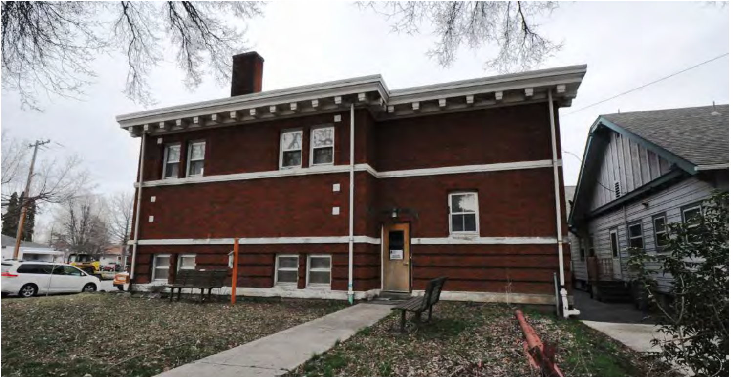
Figure 4: LaGrande Carnegie Library from the west. © Richaven Architecture & Preservation, 2020. DSC_0007.JPG.
