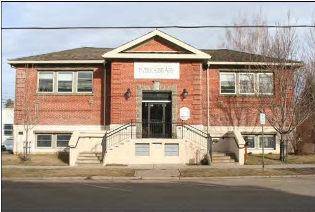
Photo 2 of 14: West façade (front), looking east.
