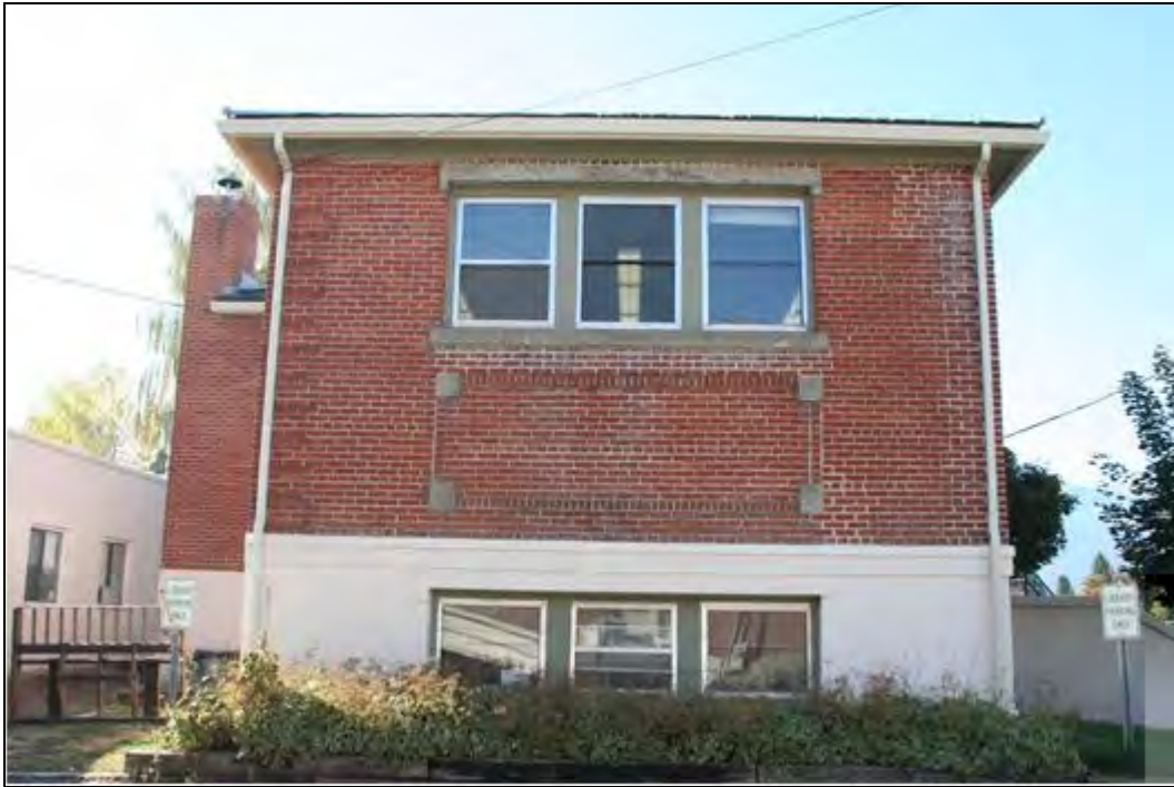
Photo 5 of 14: North façade, looking south.
