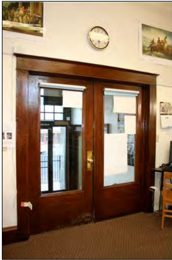
Photo 9 of 14: Entrance doors on west wall of circulation area, looking northwest.
