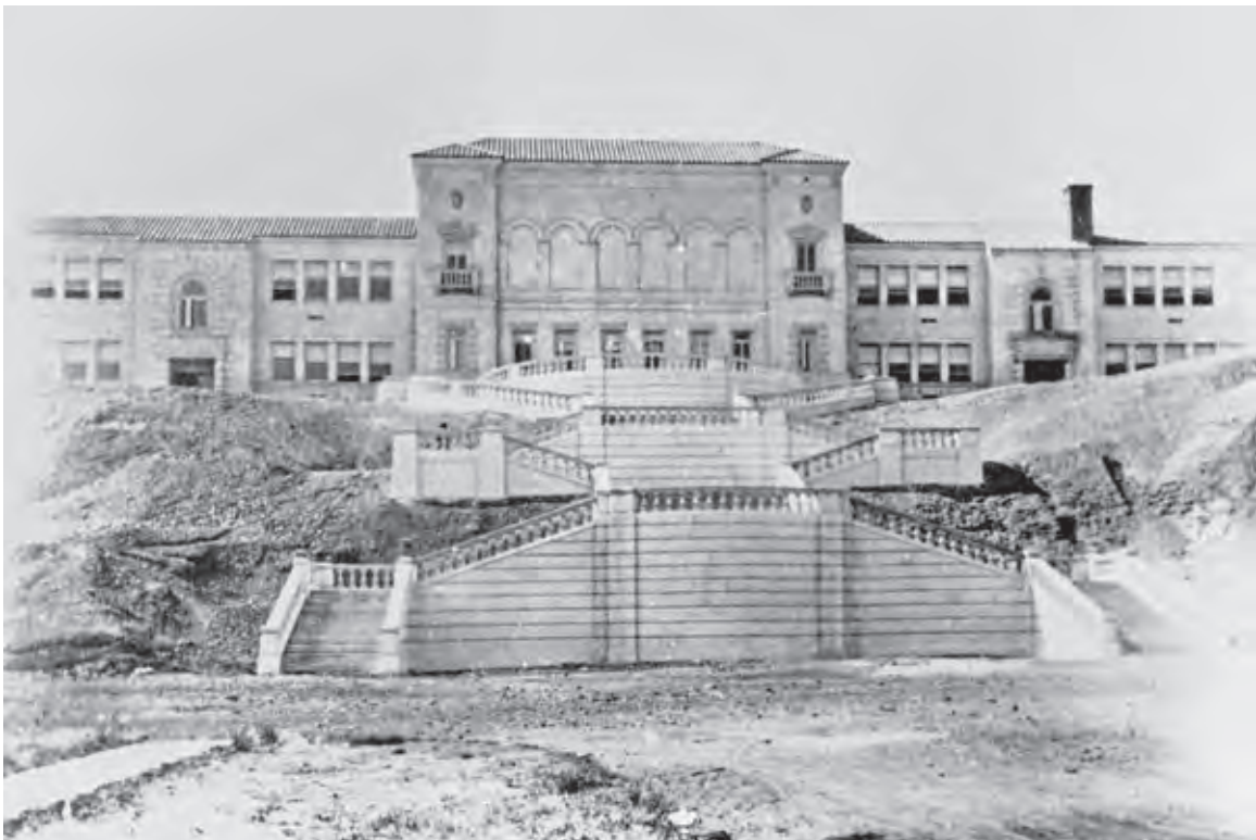
8. Grand Staircase nearly completed, 1928. North elevation, facing south. Courtesy of Eastern Oregon University Digital Archives.
