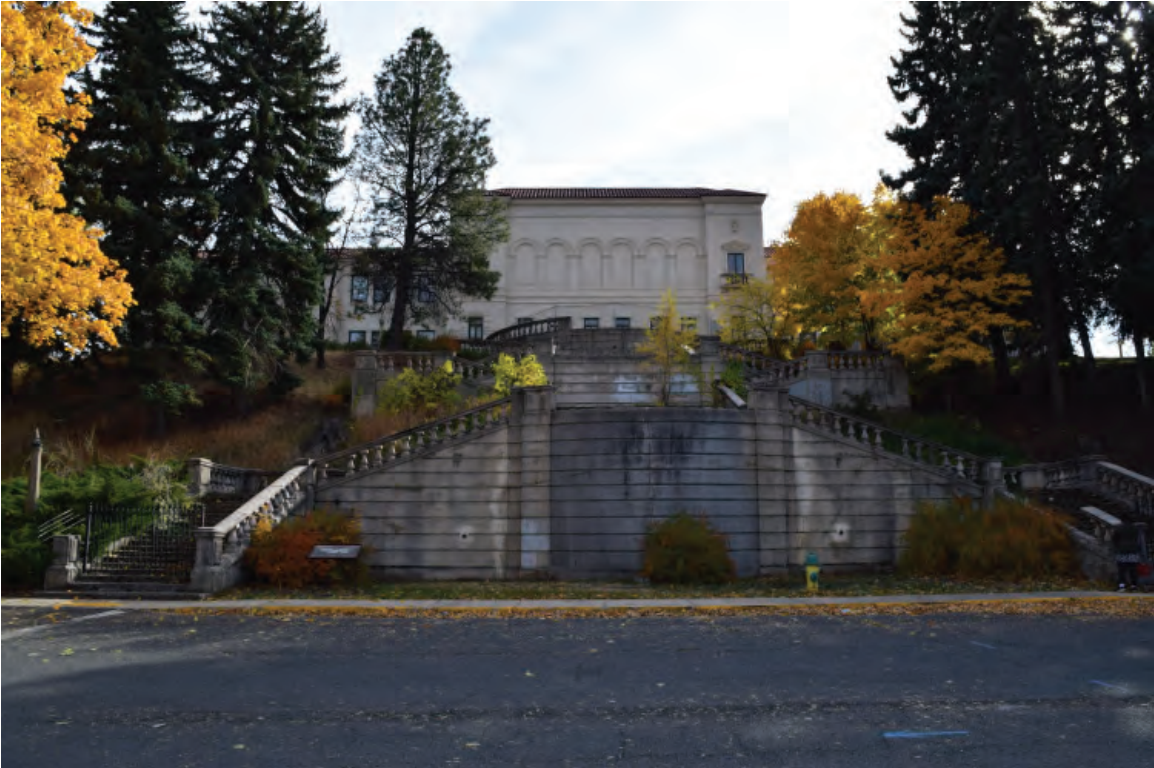
1. Grand Staircase north elevation, facing south. 10/19/2021.
