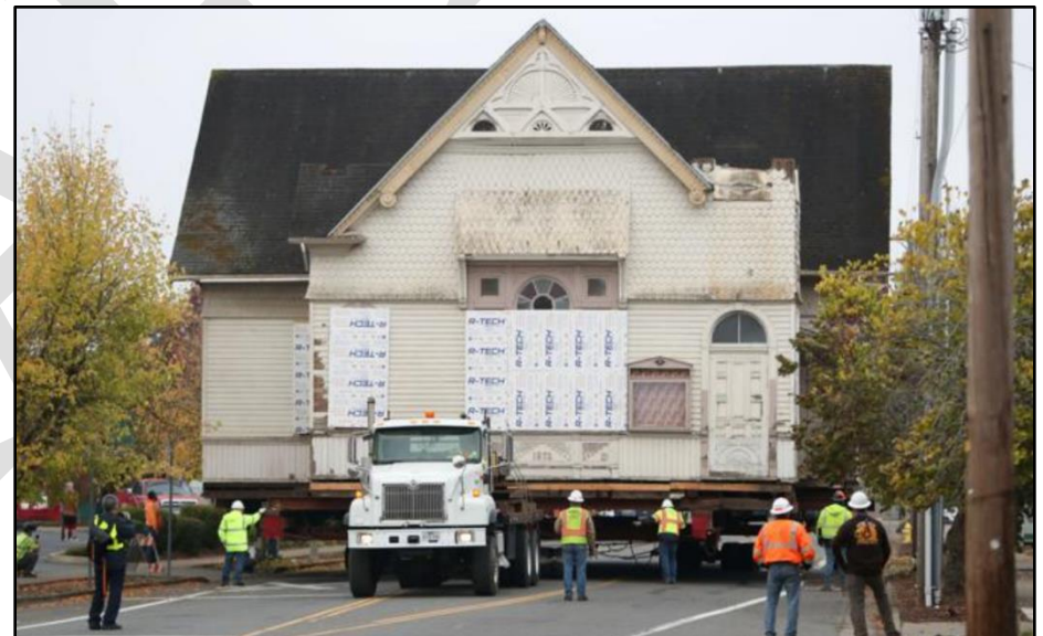
The historic Cumberland Church in Albany, Oregon, en route to its new location. The steeple was temporarily removed to facilitate the move. (Source: Corvallis Gazette-Times photo, October 2021)
