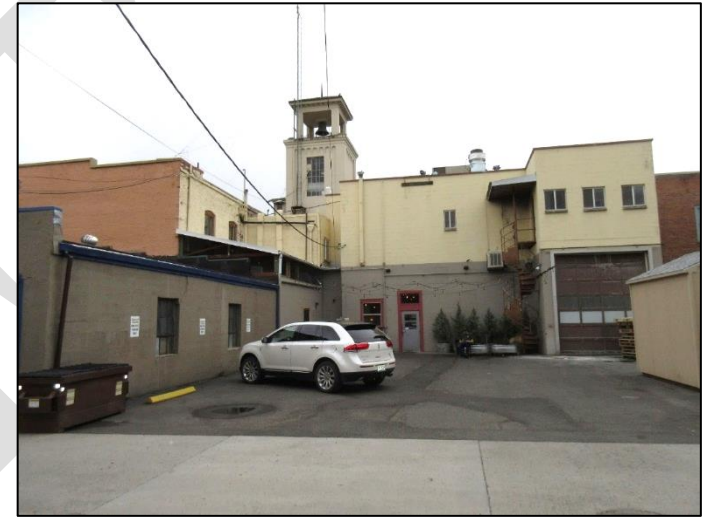
Accessory features such as planters, furniture, bollards, or trash enclosures allow for multiple uses in block interior areas and activate the alleyscape
