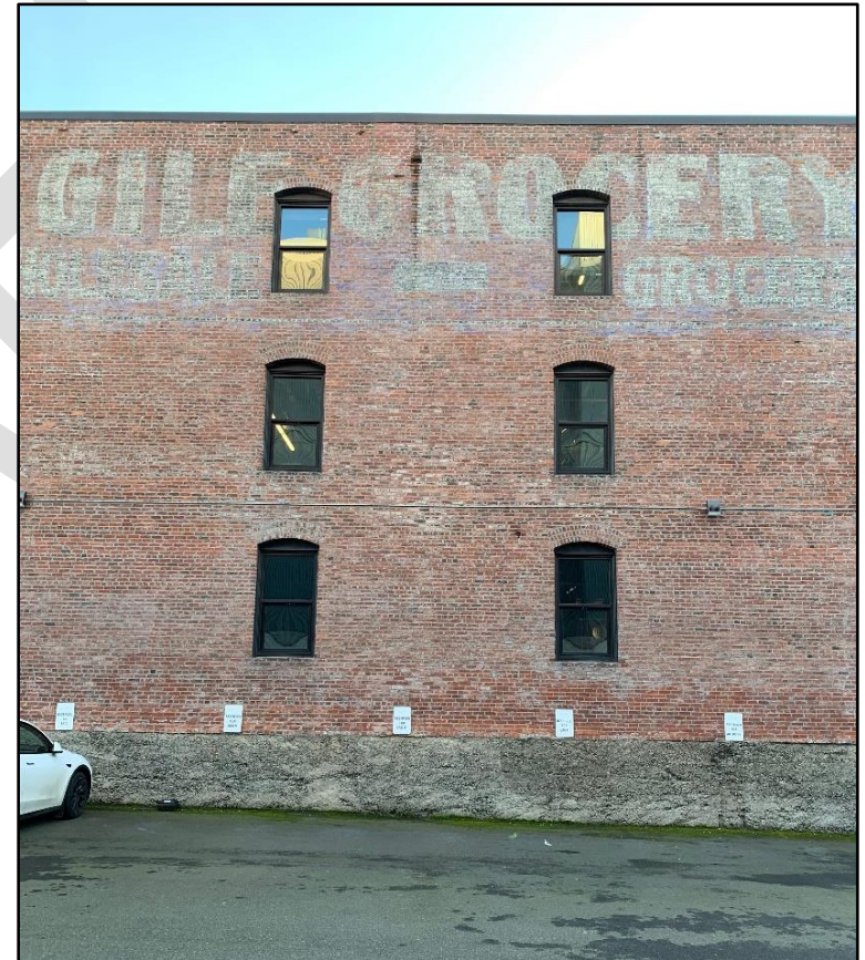
Example of aluminum windows on a rear elevation in NE Portland, OR. Note the retained "ghost" sign.
