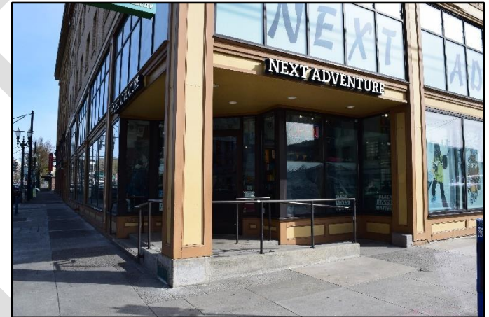
A way to retain the historic column structure and introduce a modern storefront with ADA ramp. Everyone uses the same ramp entry.
