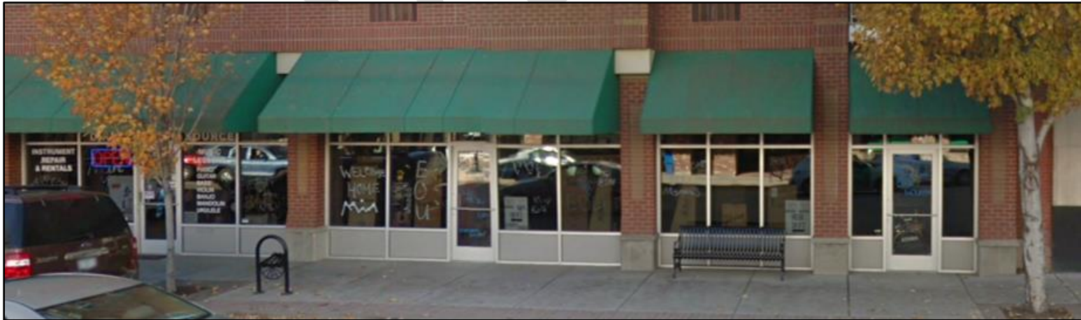
The new construction at 1206 Adams Avenue uses the historic elements of bulkhead, display windows, transom, and awning to create a historically inspired storefront with modern materials (Source: Google Street View 2018)
