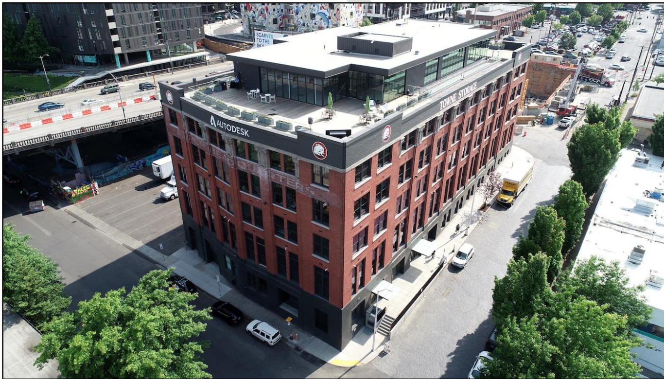
Example of a rooftop addition at the historic Towne Storage Building in Portland, Oregon. (Source: Autodesk)
