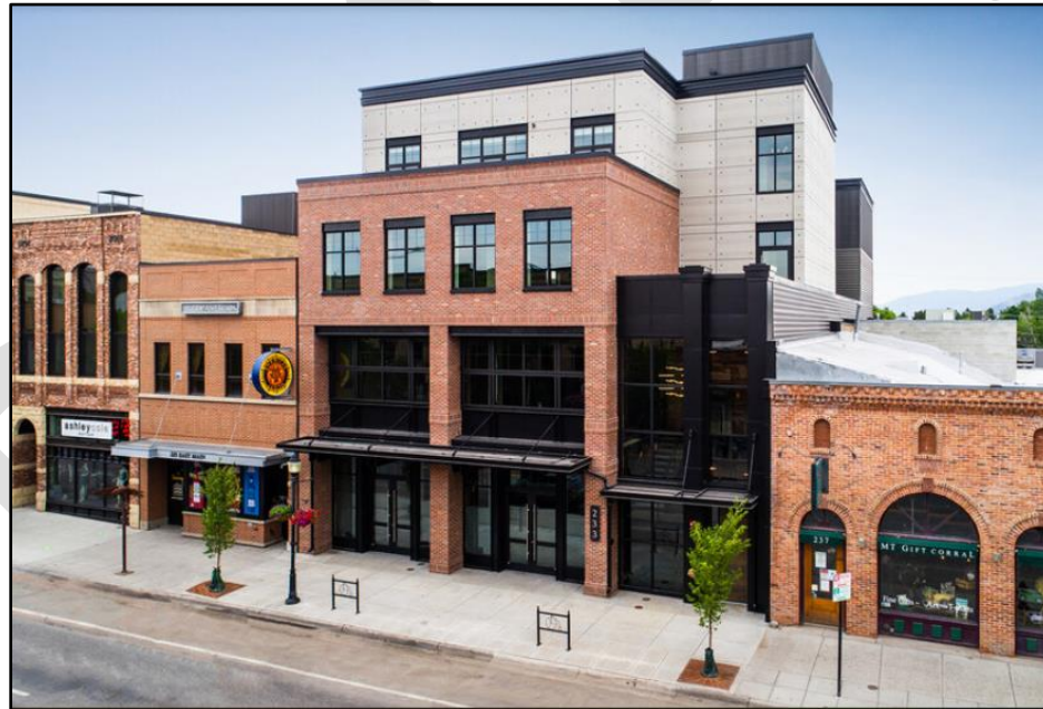
This infill development (2020) in Bozeman, MT created different volumes to break up the mass of new construction relative to the existing older buildings. The new building repairs and fills the gap in the streetwall. (Source: https://www.loopnet.com/Listin )
