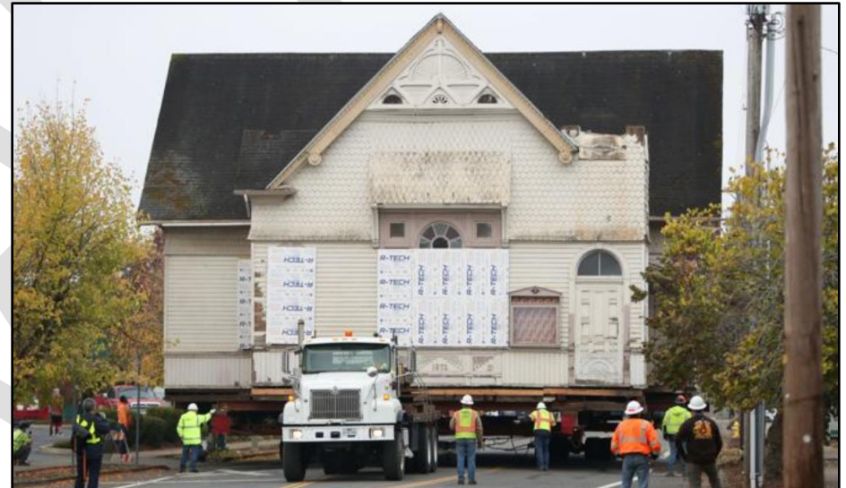
The historic Cumberland Church in Albany, Oregon, en route to its new location. The steeple was temporarily removed to facilitate the move. (Source: Corvallis Gazette-Times photo, October 2021)
