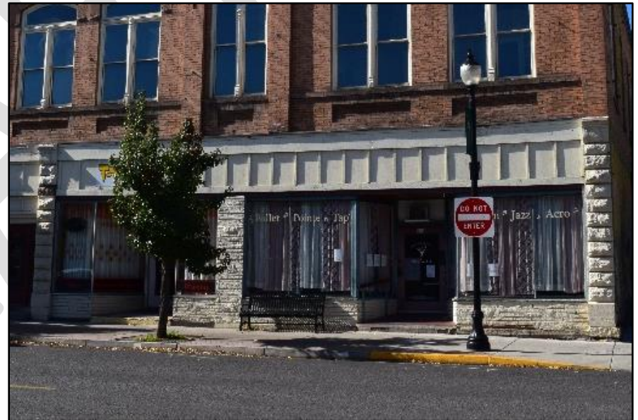
Benches, light fixtures all compatible with historic district. Other features to consider include bike lock locations, trash cans.
