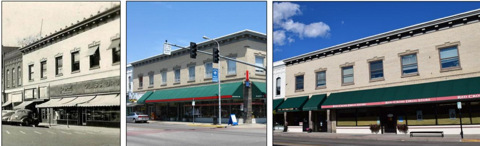
Sommer Block (1119-1123 Adams Avenue) These images show the windows and storefronts of the Sommer Block in the 1950s, 2008, and 2021. The current windows replaced inappropriate modern windows and returned the building to a more historic appearance. (Sources for left two images: http://cinematreasures.org/ , Google Street View)
