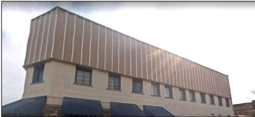
Rehabilitated upper floor of the Rogers Building at 1201 Adams Avenue with a contemporary, but compatible design around the original window openings. (Sources: Google Street View 2009 and 2015)
