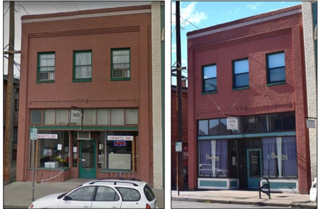
212 Fir Street is a good example of a rehabilitated storefront. Note the new panelized bulkhead beneath the storefront windows. (Source for image on left: Google Street View 2012)
