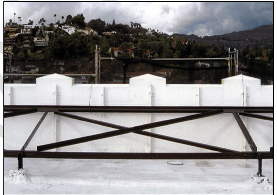
Example of parapet bracing (Source: National Park Service)
