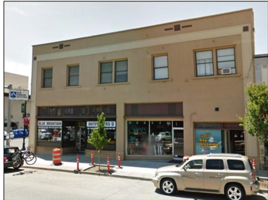
Ralston Block (1124 Adams Avenue) Note the removal of the added "fieldstone" facing and restoration of the historic stucco wall finish. (Source: Google Street View 2012 and 2015)
