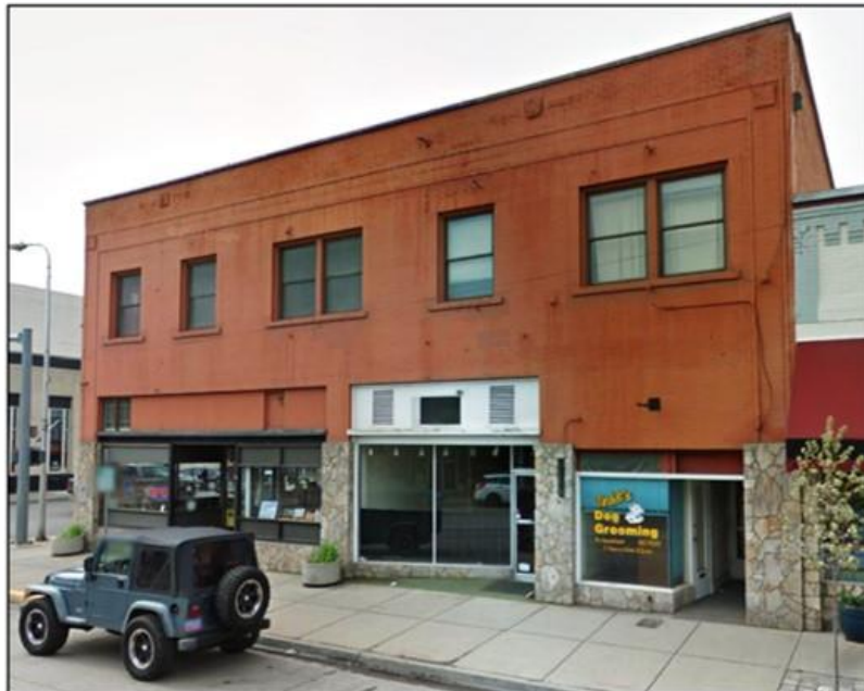
Ralston Block (1124 Adams Avenue) Note the removal of the added "fieldstone" facing and restoration of the historic stucco wall finish. (Source: Google Street View 2012 and 2015)
