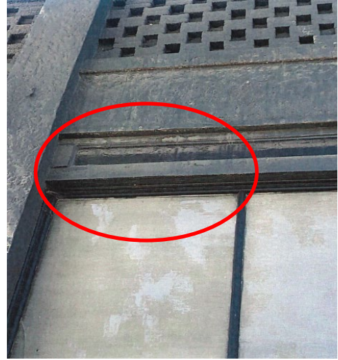
Bulkhead trim to match detail above transoms.
