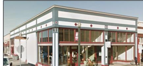
The Allen Building at 1004-1008 Commercial Street in Astoria, OR installed a historic inspired storefront. (Source: Circa 1920s Newspaper, 1989 Oregon SHPO Inventory Form, 2018 Google Streetview)
