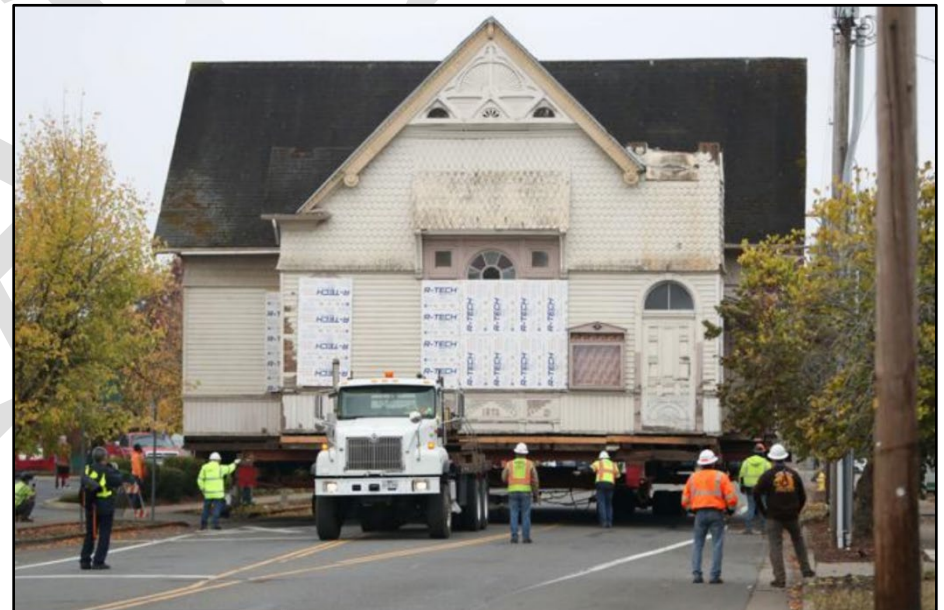
The historic Cumberland Church in Albany, Oregon, en route to its new location. The steeple was temporarily removed to facilitate the move. (Source: Corvallis Gazette-Times photo, October 2021)
