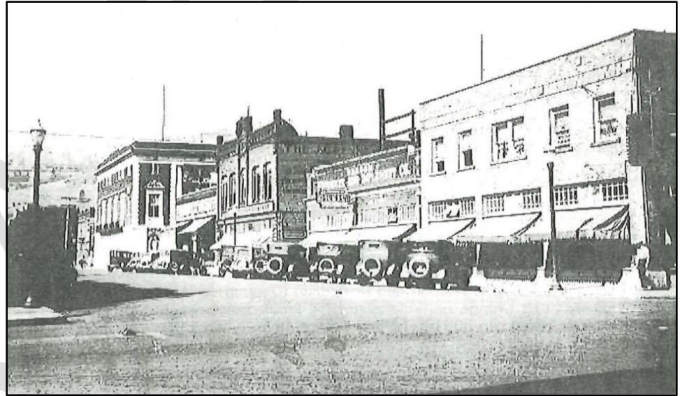
Depot Street, c. 1927, looking southwest from Adams Avenue.
