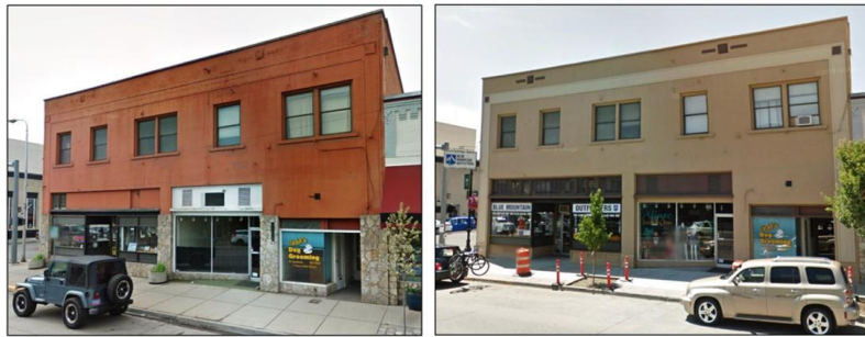
Ralston Block (1124 Adams Avenue) Note the removal of the added “fieldstone” facing and restoration of the historic painted brick wall finish. (Source: Google Street View 2012 and 2015)
