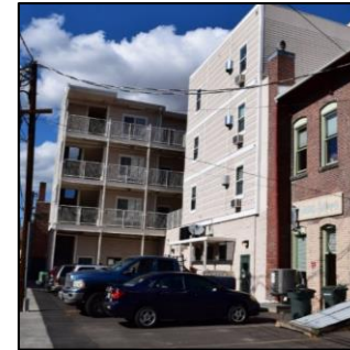
Example of materials that are allowable in the alley but would be unacceptable on the primary
