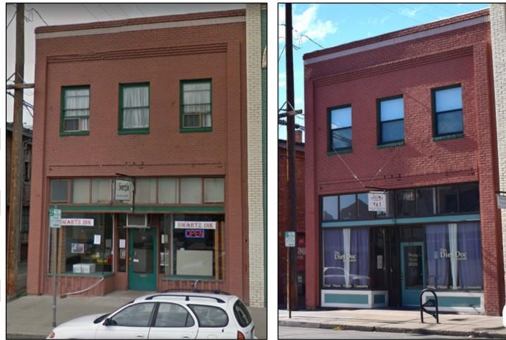
212 Fir Street is a good example of a rehabilitated storefront. Note the new panelized bulkhead beneath the storefront windows. (Source for image on left:
