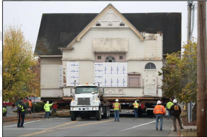
The historic Cumberland Church in Albany, Oregon, en route to its new location. The steeple was temporarily removed to facilitate the move. (Source: Corvallis Gazette-Times photo, October 2021)
