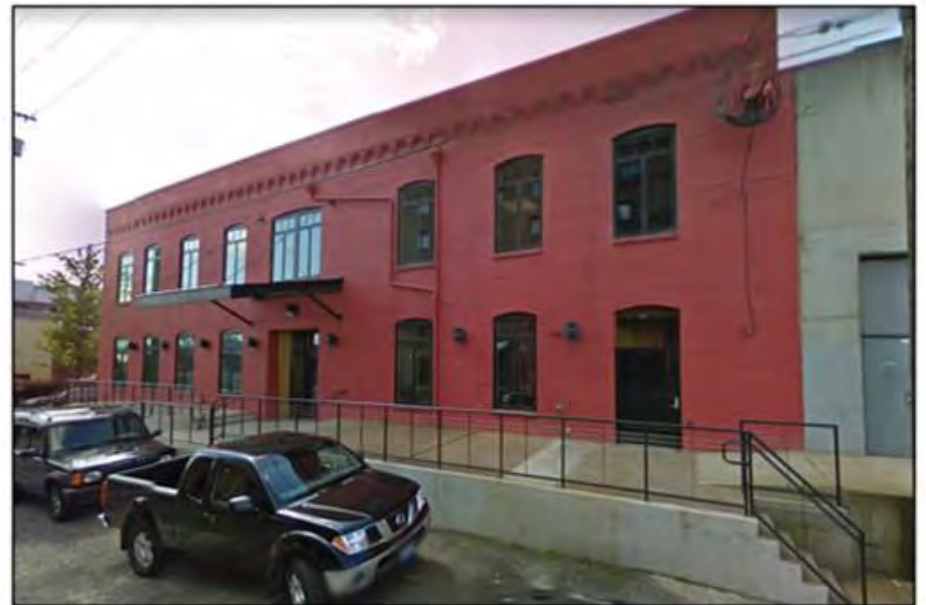
This former warehouse building was rehabilitated for a new use circa 2008. Alterations included the replacement of the small loading dock windows with larger windows. A full storefront bay expression would have conveyed the wrong “story” about the building’s original use. This style of rehabilitation could be applied to buildings along Jefferson Avenue. (Source for image on left: c.1980 City of Portland Historic Resource Inventory) (Source for image on right: 2009 Google Street View)
