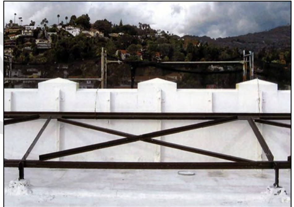
Example of parapet bracing as seen from the roof (Source: National Park Service)
