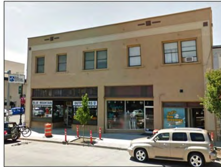
Ralston Block (1124 Adams Avenue) Note the removal of the added “fieldstone” facing and restoration of the historic painted brick wall finish. (Source: Google Street View 2012 and 2015)
