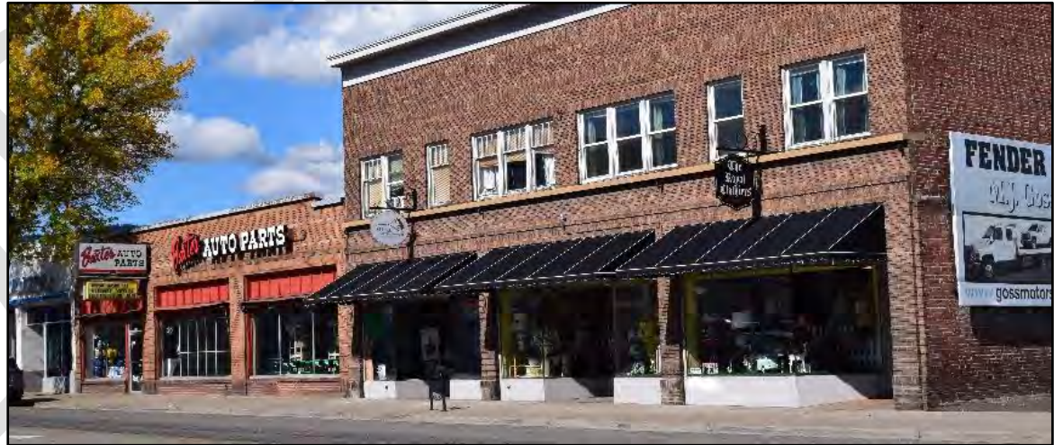
A variety of sign types are visible in this image, including blade signs, mounted wall signs, and internally illuminated letter signs. All are placed for pedestrian use and are no larger than historic building features at the ground level.
