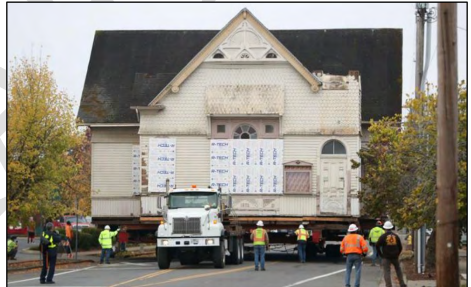
The historic Cumberland Church in Albany, Oregon, en route to its new location. The steeple was temporarily removed to facilitate the move. (Source: Corvallis Gazette-Times photo, October 2021)
