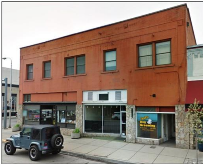
Ralston Block (1124 Adams Avenue) Note the removal of the added “fieldstone” facing and restoration of the historic painted brick wall finish. (Source: Google Street View 2012 and 2015)
