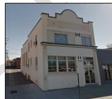
Salvation Army Building, Fir St. (image Google streetview)
