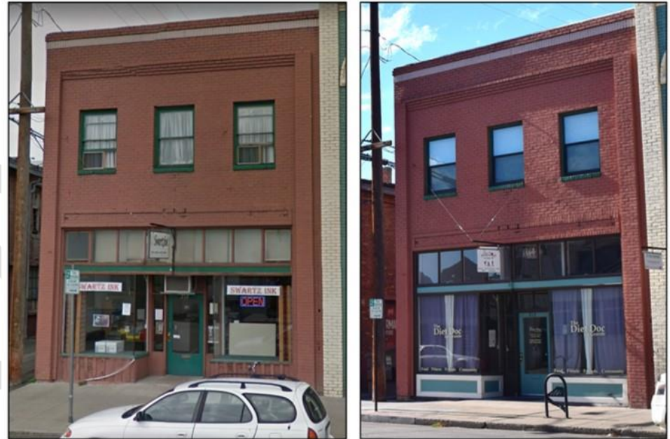
212 Fir Street is a good example of a rehabilitated storefront. Note the new panelized bulkhead beneath the storefront windows. (Source for image on left:
