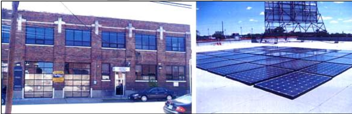
Using flat or low-slope solar panels is a simple way to limit visibility. (Sources: National Park Service: https://www.nps.gov/tps/sustainability/new-technology/solar-on-historic.htm )
