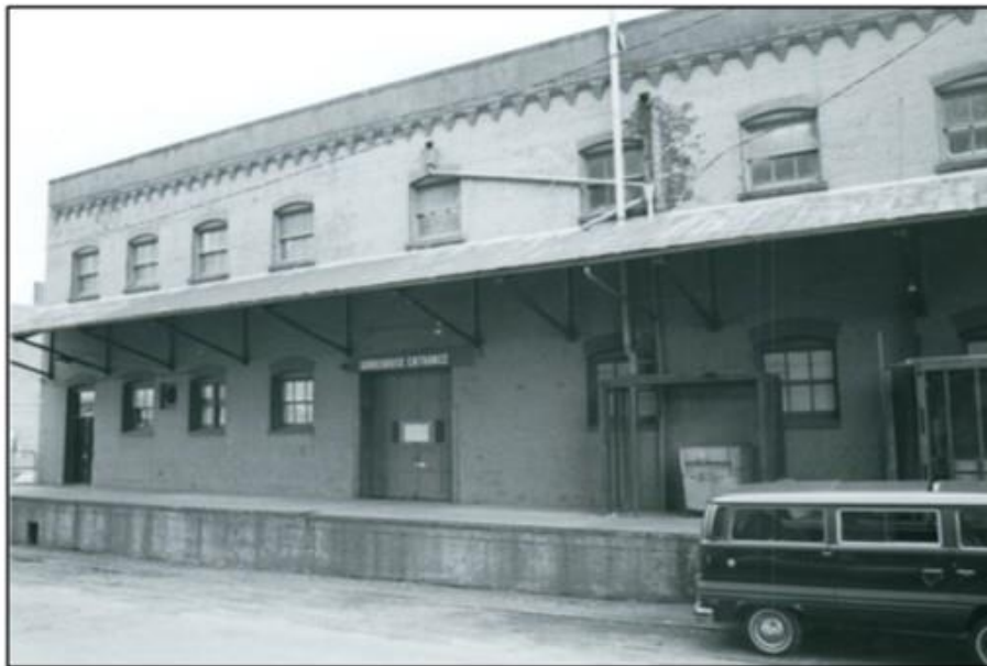
This former warehouse building was rehabilitated for a new use circa 2008. Alterations included the replacement of the small loading dock windows with larger windows. A full storefront bay expression would have conveyed the wrong “story” about the building’s original use. This style of rehabilitation could be applied to buildings along Jefferson Avenue. (Source for image on left: c.1980 City of Portland Historic Resource Inventory) (Source for image on right: 2009 Google Street View)
