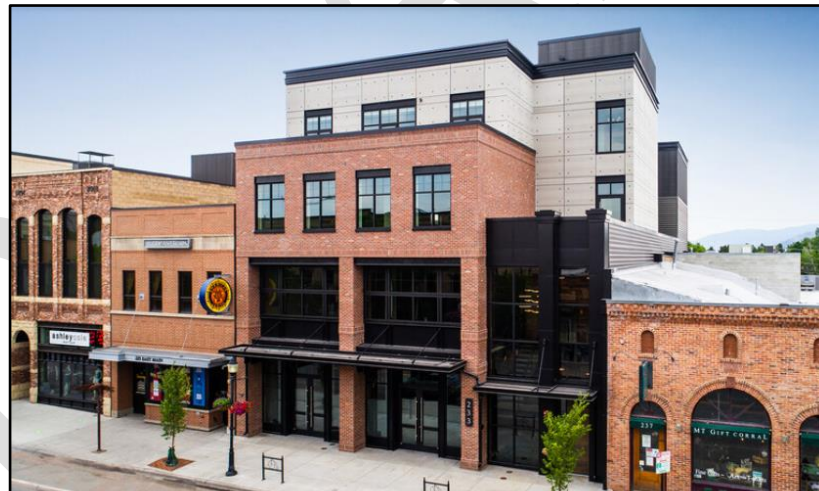
This infill development (2020) in Bozeman, MT created different volumes to break up the mass of new construction relative to the existing older buildings. The new building repairs and fills the gap in the streetwall. (Source: https://www.loopnet.com/Listin )
